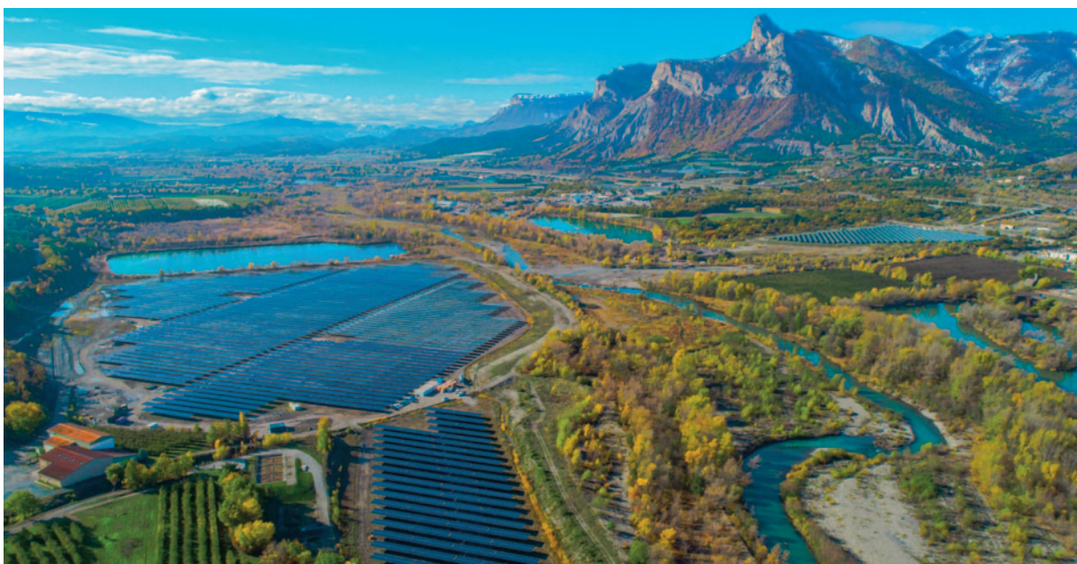
15 MW, Curbans, France.
