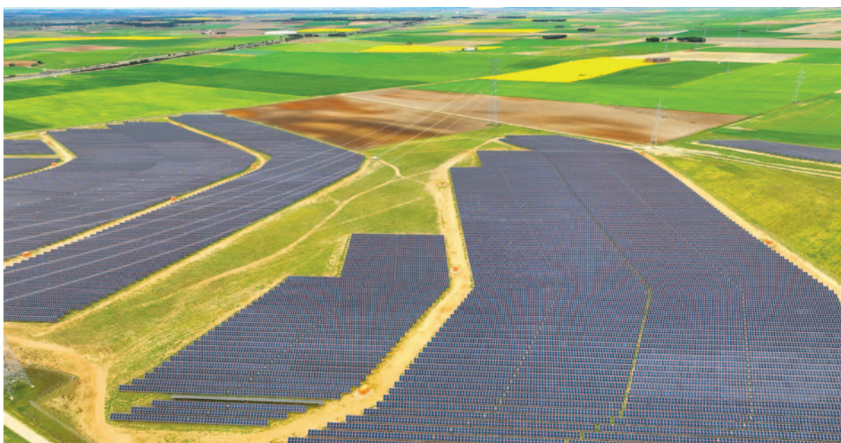
41.7 MW, Tordesillas, Spain.
