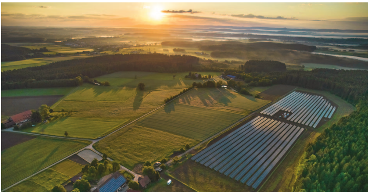
7.27 MW, Pfaffenweiler, Germany.
