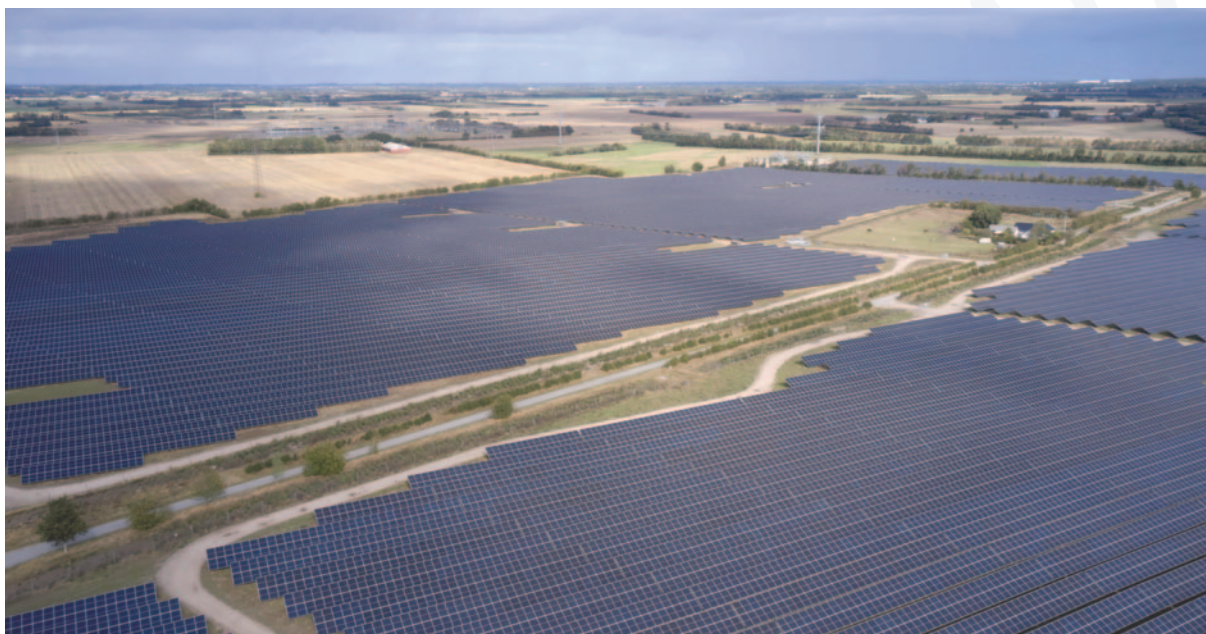
The 304 MWp Kassø PV plant was grid connected in 2022 to the 165 kV side of one of the main TSO transformer stations in the southern part of Denmark. It is constructed with half a million bifacial modules. In 2023 it will be connected to a 50 MW electrolyser and the world's largest e-methanol plant capable of producing 30,000 tons of green shipping fuels per year.
